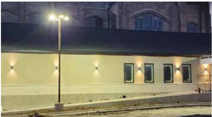
Exterior lighting now illuminates the east side of the Gathering Center in addition to our parking lot.
