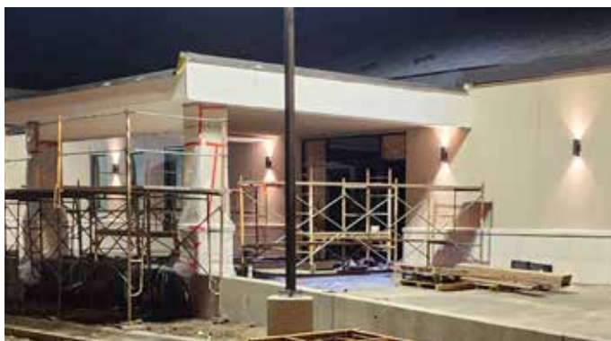
Our covered entrance takes shape over our newly poured ramp.
